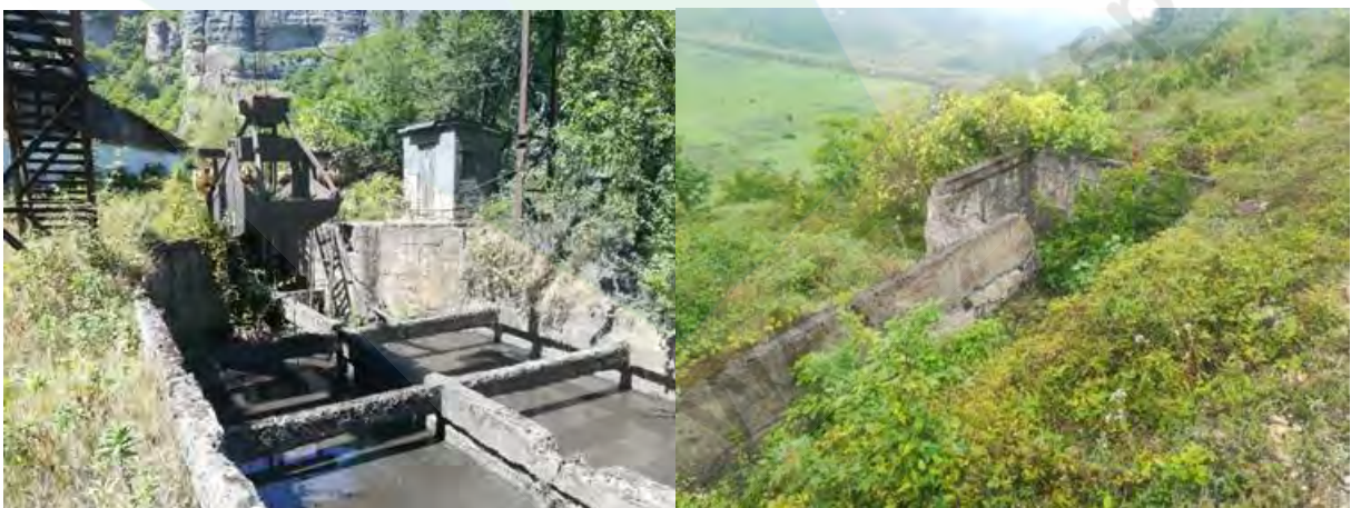
Figure 22: Abandoned tailing pond (left) and tailing canal (right).
