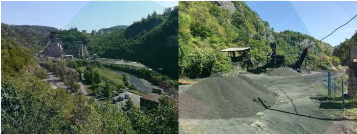
Figure 18: Mn ore processing plants – principal processing plant governed directly by Georgian Manganese (left), small scale processing plant allegedly governed by a subcontractor (right)
